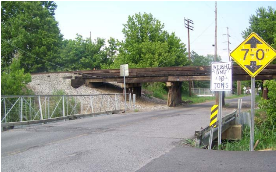
Exhibit 6: KY-1826 approaching Project Bridge looking east
