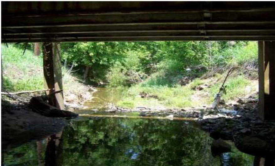
Exhibit 13: KY-1826 Project Bridge looking Downstream
