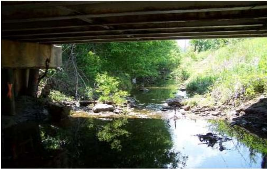
Exhibit 12: KY-1826 Project Bridge looking Upstream
