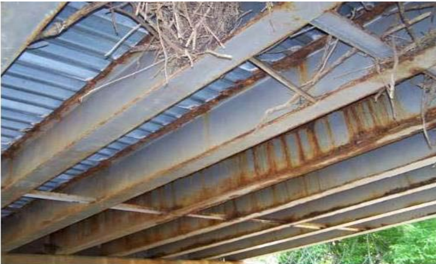
Exhibit 14: KY-1826 Project Bridge looking on Steel Beams
